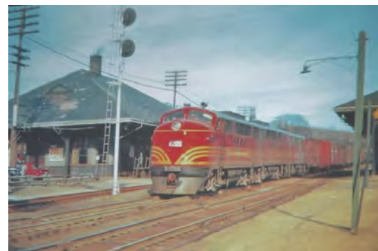
One of the diesel engines that replaced the old steam engine. Photo from B&M Railroad Historical Society.
