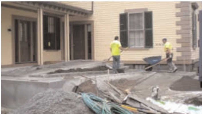
Walkway prepped by Cataldo Landscape crew for pouring cement apron and sidewalk. Photo by Barbara Murray.
