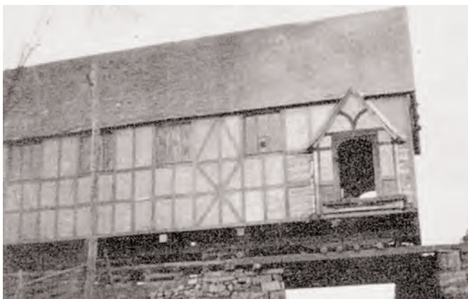
On September 27, 1904, the former Groton School chapel was horse-drawn on rollers down Farmers Row and West Street across a narrow bridge over the railroad tracks to its new home at 297 Main Street. Photo courtesy of Sacred Heart Church.
