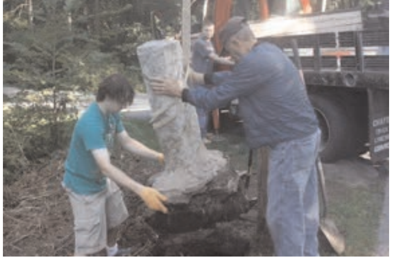
Resetting by hand and crane.
