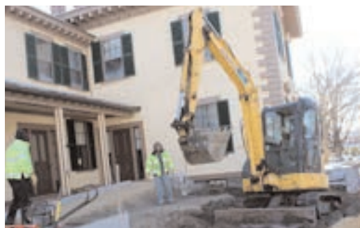
Tiago (with rake) and crew compact and sculpt soil and sand dropped from the bucket of a front-end loader. Concrete pavers finish the surface of the new ADA accessible walkway at the side of Boutwell House.
