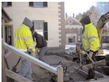
Tiago (with rake) and crew compact and sculpt soil and sand dropped from the bucket of a front-end loader. Concrete pavers finish the surface of the new ADA accessible walkway at the side of Boutwell House.
