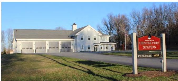
New Center Fire Station opened June 18, 2014, on Farmers Row – a state-of-the-art facility ready to serve the citizens of Groton for years to come. Photo by C. David Gordon.
