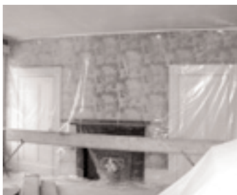
From left: dining room protected with plastic sheeting, office insulated, wallboard installed, replastering done.
