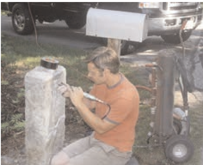
Reset milestone is re-engraved prior to being “drawn in black.”
