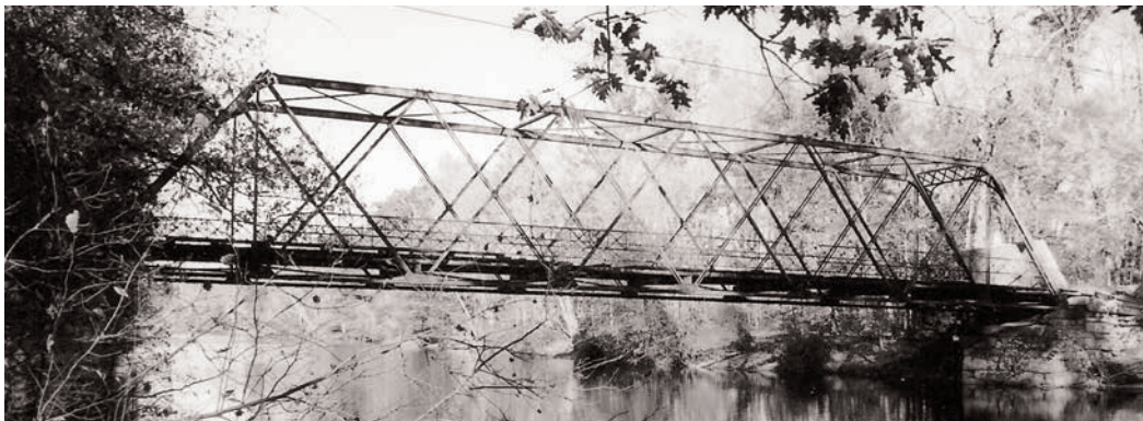
The present Fitch's Bridge, graciously suspended over the Nashua River since 1874, but condemned and off-limits even to foot travel since 1966, will be removed and replaced this summer by a truss bridge with weathered steel finish designed to resemble the old bridge and thus reflect part of its heritage. Photo by Russell Harris.
