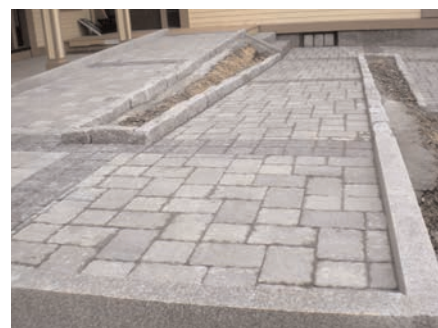
Tiago (with rake) and crew compact and sculpt soil and sand dropped from the bucket of a front-end loader. Concrete pavers finish the surface of the new ADA accessible walkway at the side of Boutwell House.
