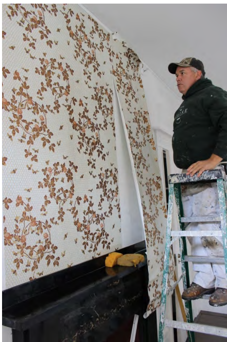
With consummate skill Dan Lowney applies custom wallpaper to the Boutwell House dining room walls. Photo by C. David Gordon.
