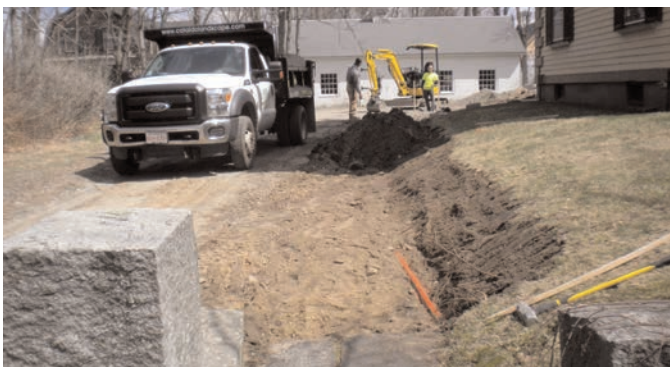
Making way for the new sidewalk. Photo by Barbara Murray.
