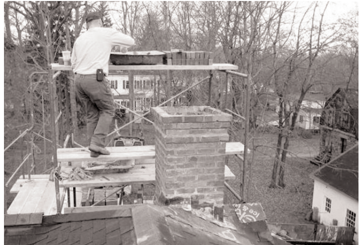
New kitchen chimney under construction. Photo by Al Collins
